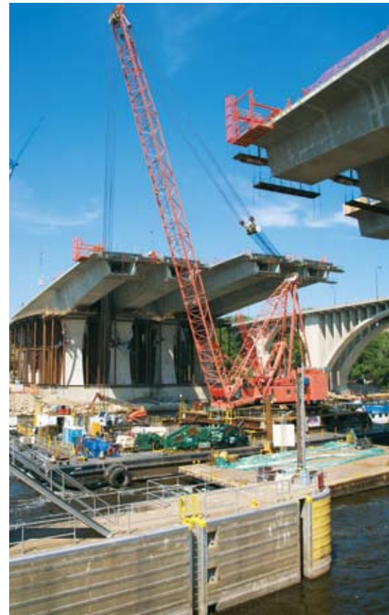
Precast segments weighing up to 200 tons were erected quickly. Photo: © FIGG.
